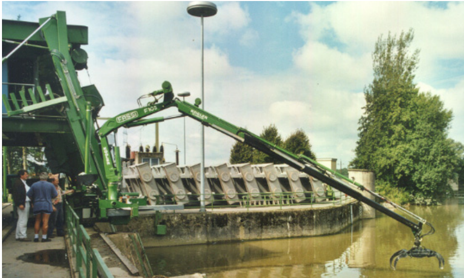
Crane with timber grab TC Gralla
