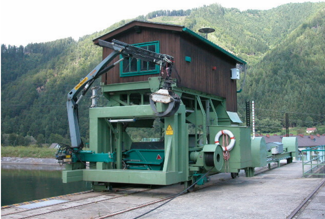
TC Pernegg with crane and container wagon
