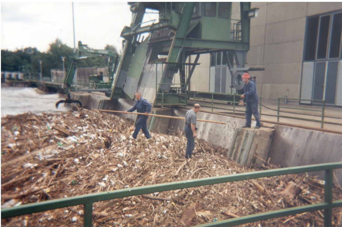
Accumulated debris & driftwood in Gralla (after refurbishment of the TC)
